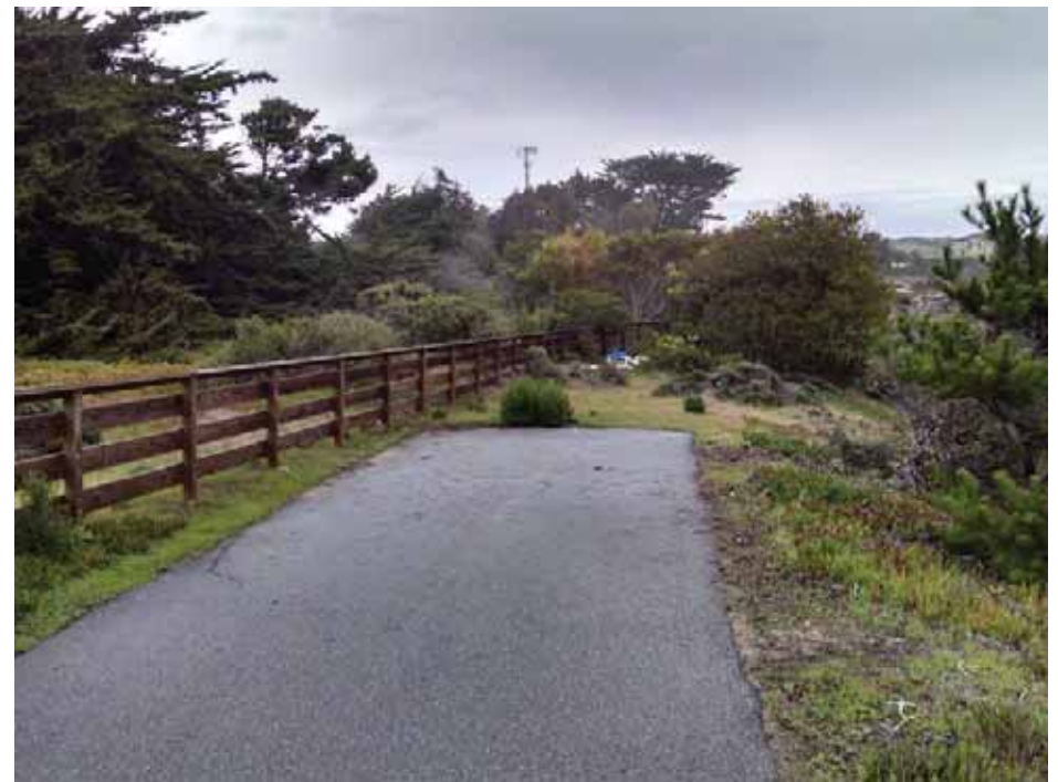
Photo 3. View of proposed replacement lift station site facing north.
