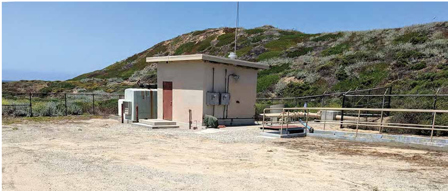
Photo 1. View of existing Fort Ord Lift Station.
